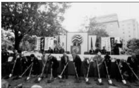
Turning the first shovels of dirt was a task for many hands at the groundbreaking ceremonies.
